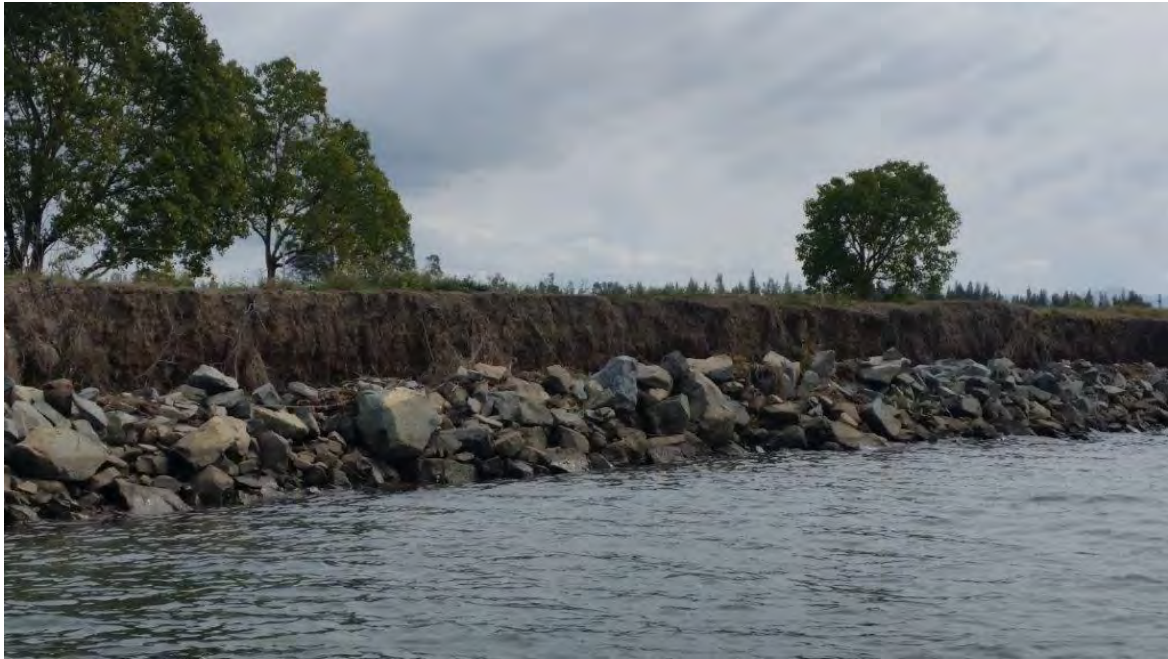
Photograph 4 Rock revetment and fencing on Jones Island (205) to protect bank from further erosion
